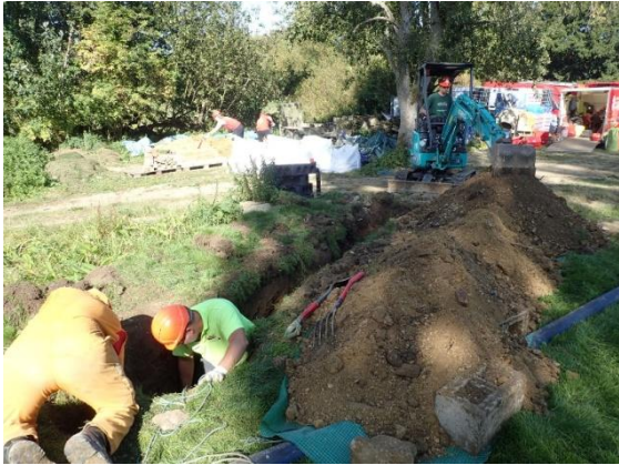
Pipework trench. Photo: Tim Lewis
