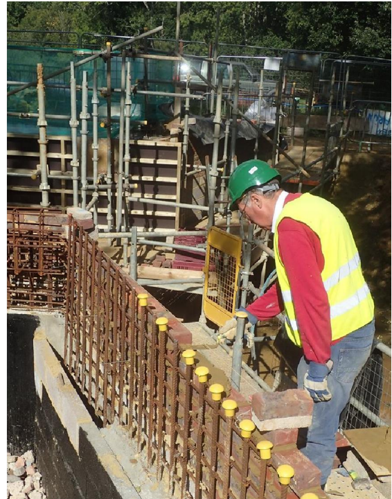
Whilst the brickies wanted 'just one more load' of muck.
