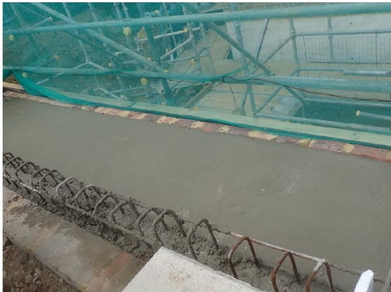
We finished the 4m3 pour in about three hours!
